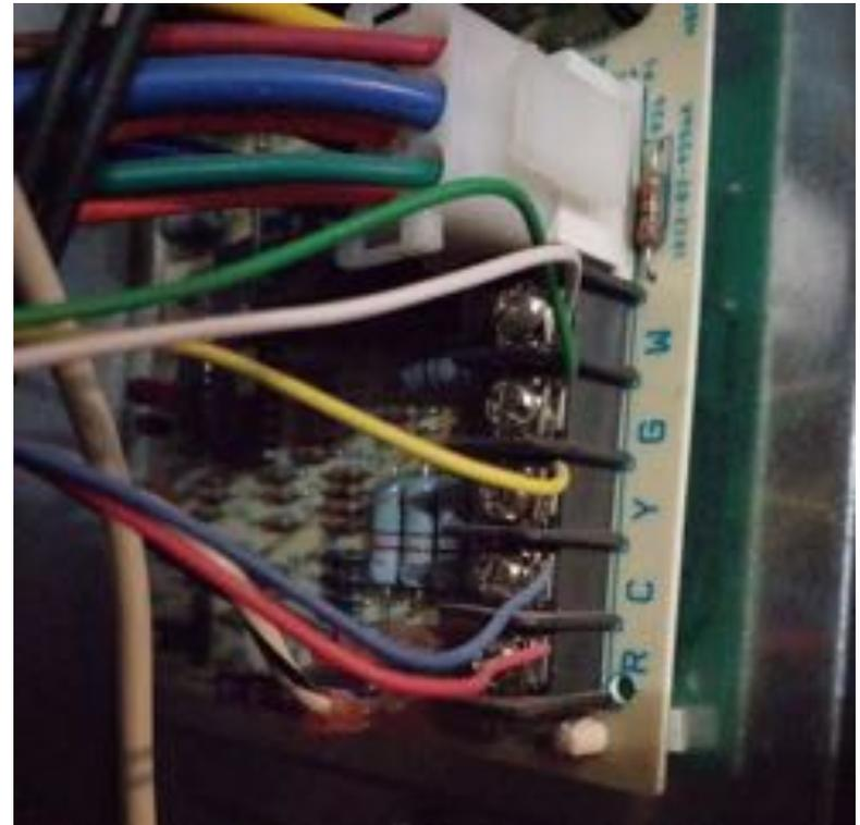
The control board should look similar to the picture above. The control board has wires with the same colours and thickness as the wires on the thermostat. You will also find labelings similar to those at the thermostat.
