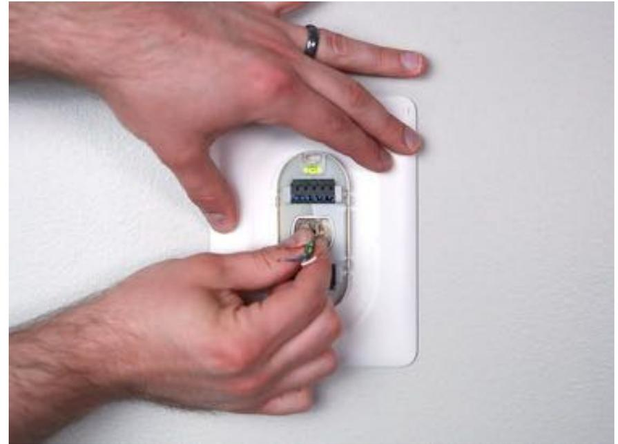
Use the included drywall anchors and screws to mount the back panel to the wall. Keep centering the bubble on the built-in level to make sure your thermostat is in alignment.
