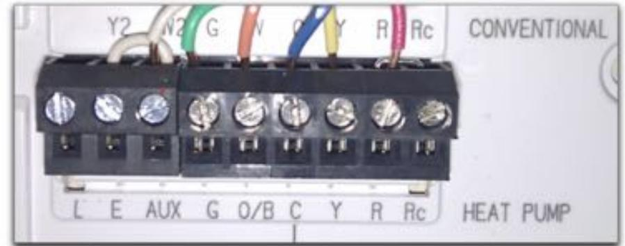
2. Unused wire(s): It is best to identify if the wire is used at the control panel as well. If the wire is being used at the control panel, please label it clearly with the included label. If it is not being used, label your unused wire with the empty sticker label.
